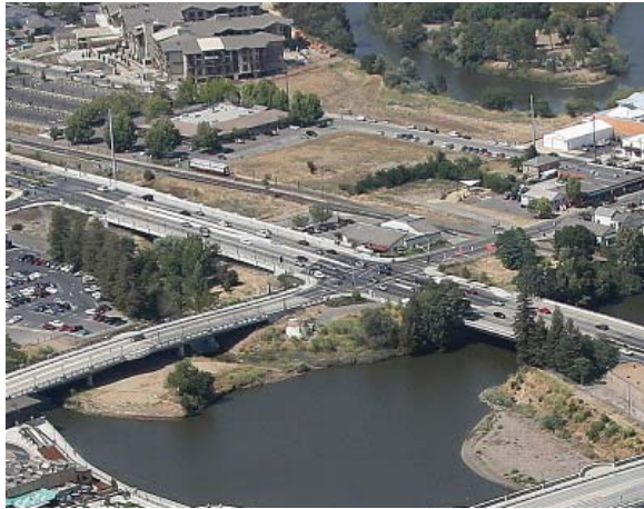
The Oxbow Bypass project is scheduled to be completed in 2013.
